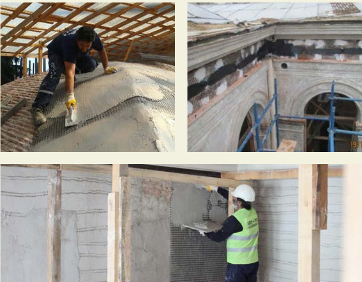
Figure 3: Examples of the retrofitting of heritage structures using textile-reinforced mortar
